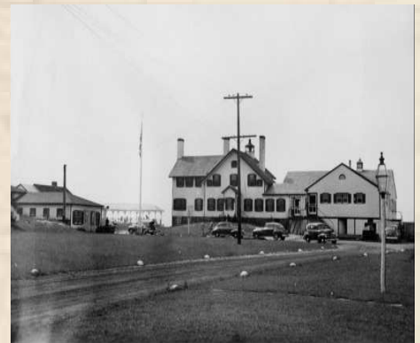
June, 1945 A new dining room and kitchen were constructed on a steel frame with walls designed to break-away in the event of hurricane.
