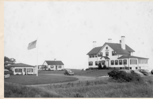
The beginning of Lighthouse Inn 1938
